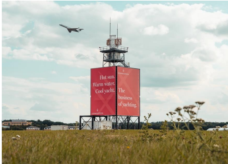
The construction of the radar tower advertisement is now complete
